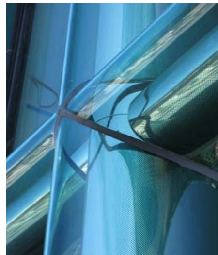
Figure 4 – Typical Mullion Intersection
